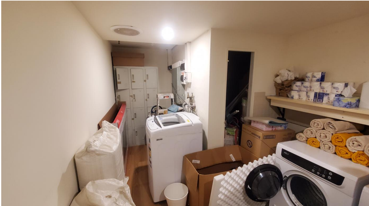
Figure 11: Laundry located at basement level
