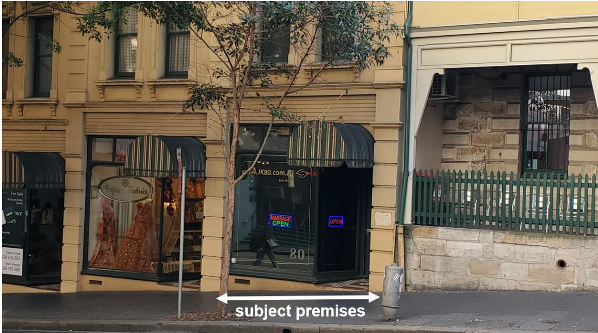
Figure 3: Subject premises (No. 80) as viewed from Erskine Street facing northwest
