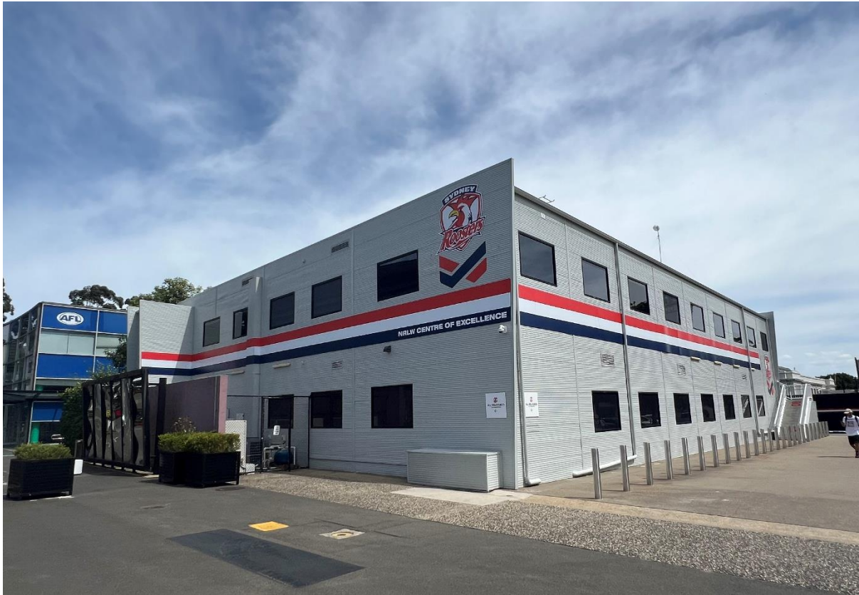
Figure 9: View of the existing Sydney Roosters Headquarters, which is situated between Area 1 and Area 2
