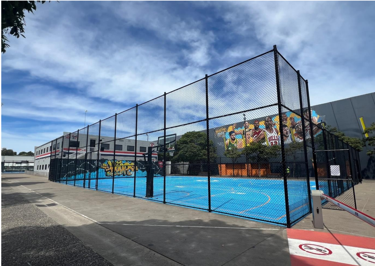
Figure 3: View of Area 1 (basketball court) looking south-east
